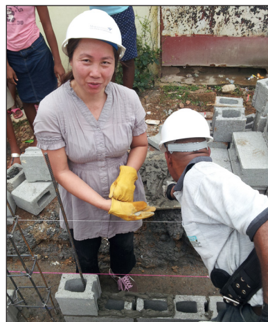
Terri Yan working at the construction site in The Dominican Republic
